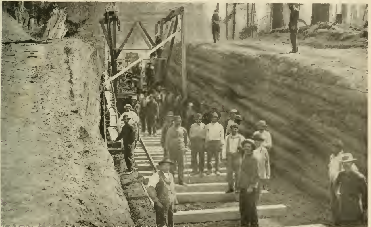
THE NORTHERN PACIFIC PENINSULAR EXTENSION—LAYING TRACK IN AN UNFINISHED CUT.
